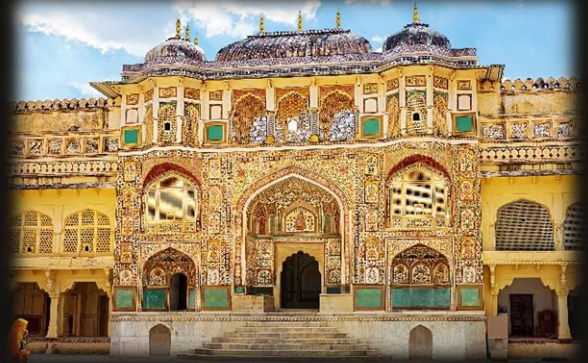
Amber Fort entrance point
